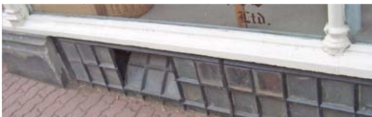
Example of glass blocks stall riser, 1920's.
