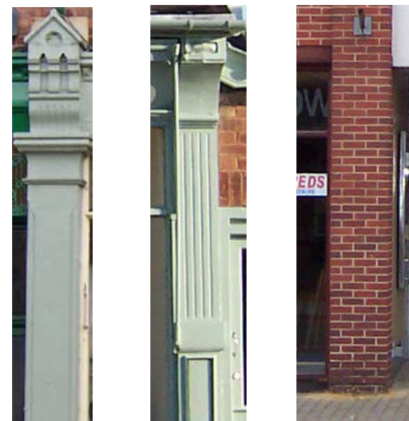
A stone, timber and brick pilaster
